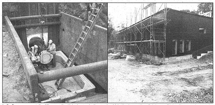
Left: Crews connect the Minneapolis 48-inch supply line to the 24-inch pipe to New Brighton. Right: Construction on the distribution control station building, which will house the permanent booster pumps.
