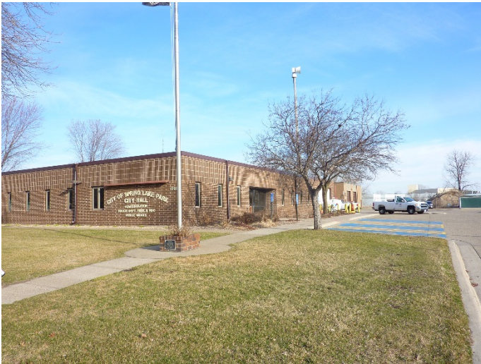
Figure 4. Flag pole and emergency siren near main entrance
