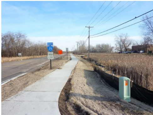
Figure 12. New sidewalk along Central Ave NE
