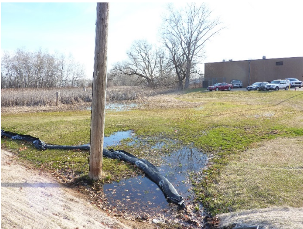
Figure 9. Ponding in the Wetland Area
