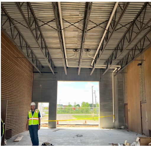
New cold storage space between the main and North garages—June 14, 2024.
