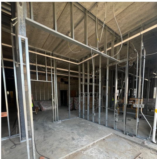
Framing in the new Police Department area—June 14, 2024.
