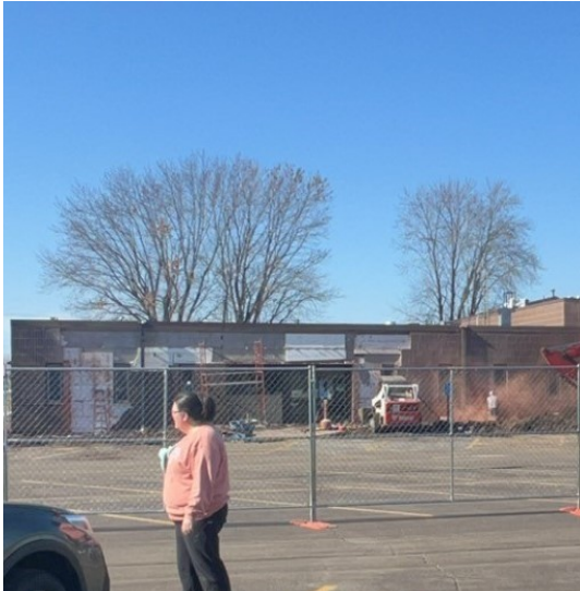
Bricks being removed from the front of the building —February 26, 2024.
