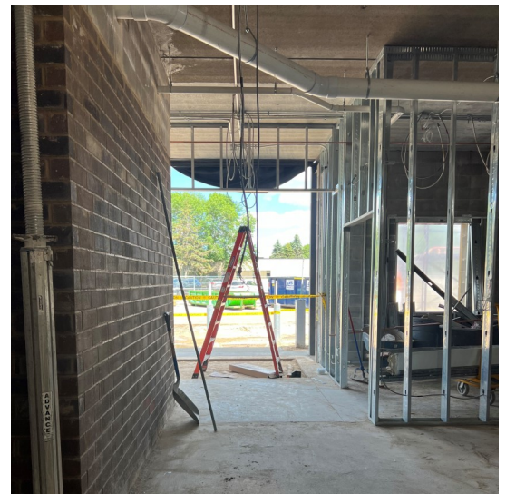
New entrance for Parks & Recreation and Administration framing—June 14, 2024.
