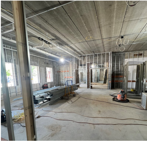
Front portion of the multi-purpose room— June 14, 2024.
