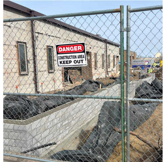
Brick work for the new addition—March 21, 2024.
