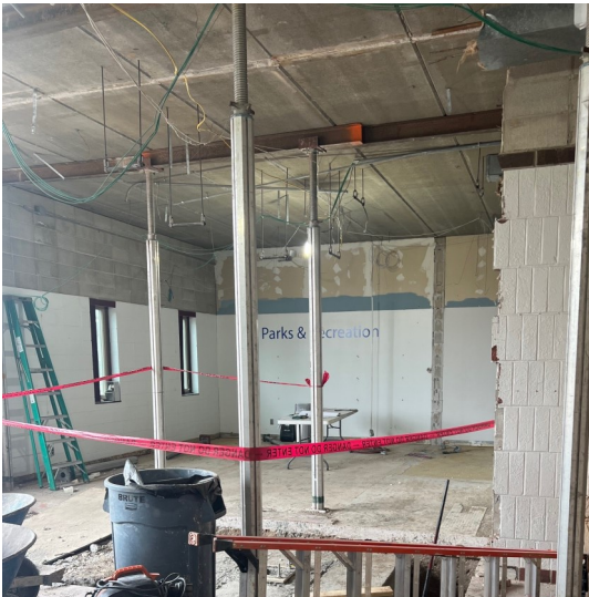
Parks and Recreation Office demolition—April 1, 2024.
