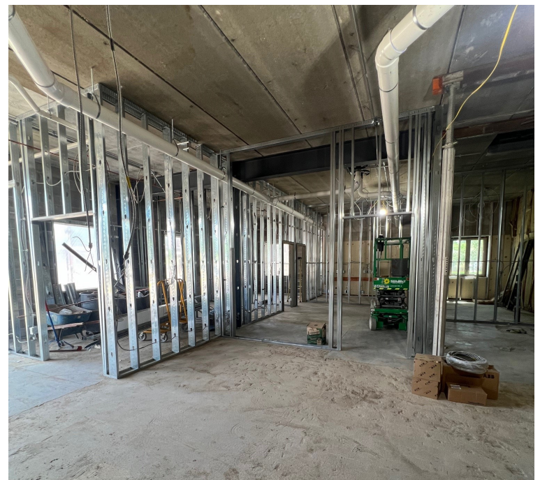
Framing of the Parks and Recreation area—June 13, 2024.
