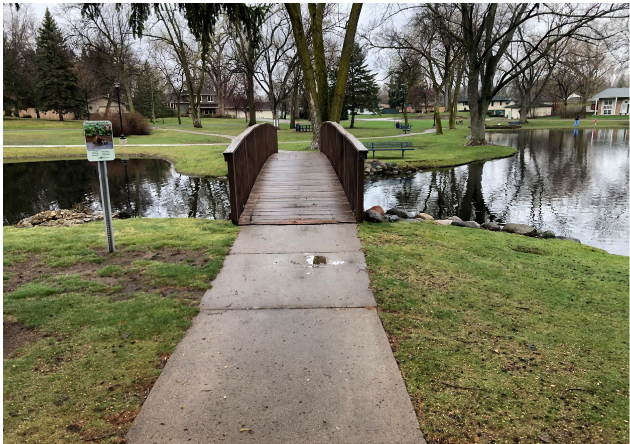
Bridge crossing over pond
