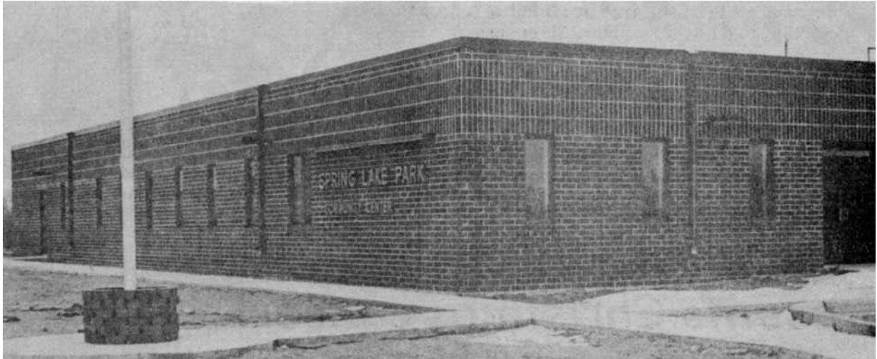
The new Spring Lake Park Community Center 1977.
